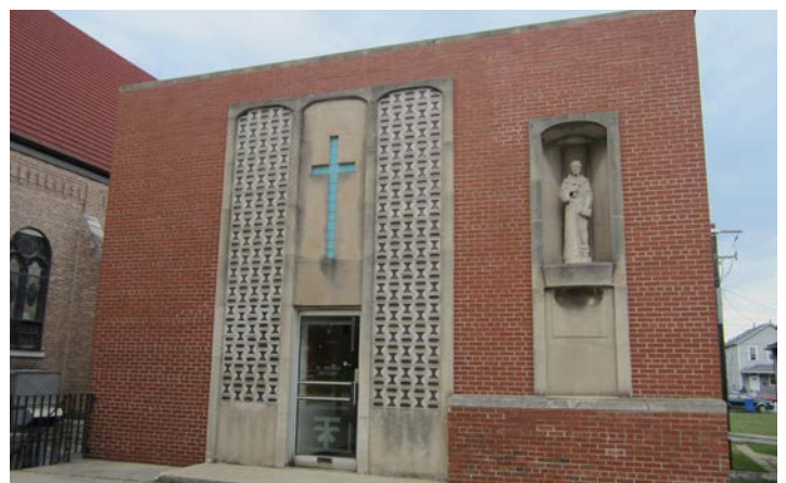
EXTERIOR RECTORY BUILDING
