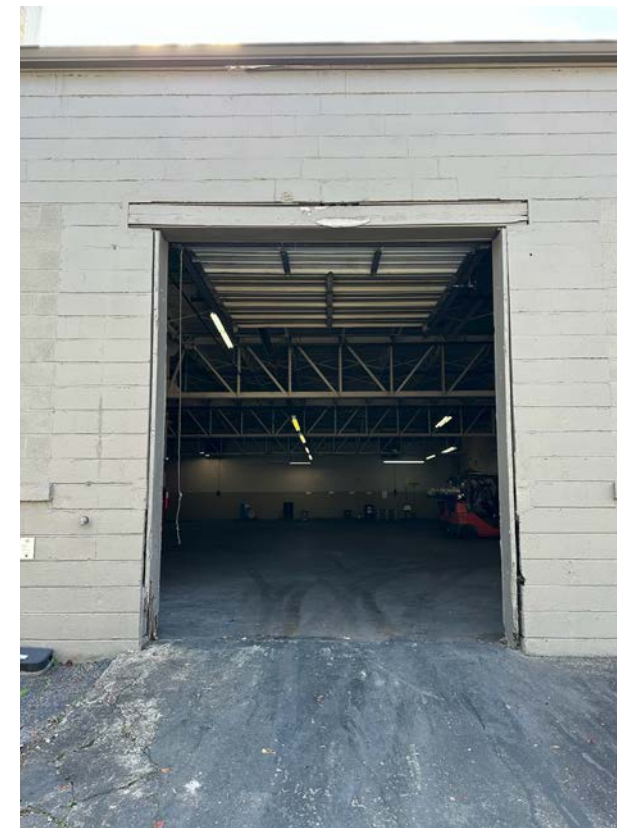
Drive In Overhead Door
